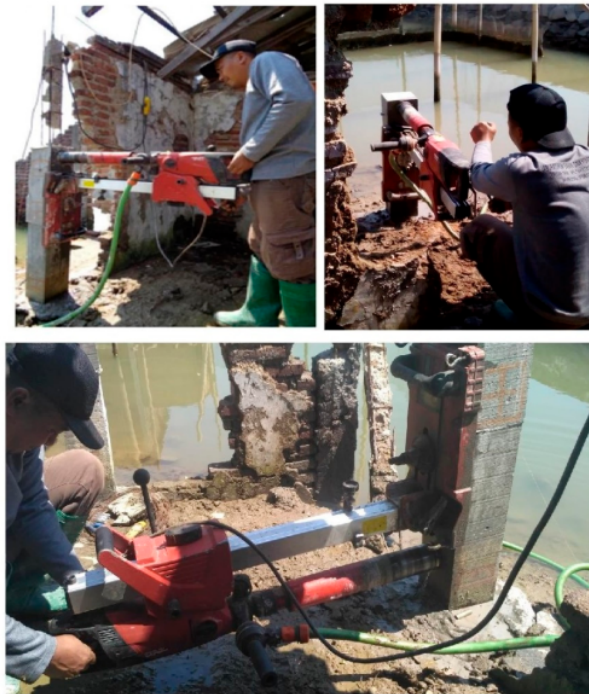
Figure 18. Core Drill method of retrofitted and control columns conducted to obtain samples used for the compressive strength test.
