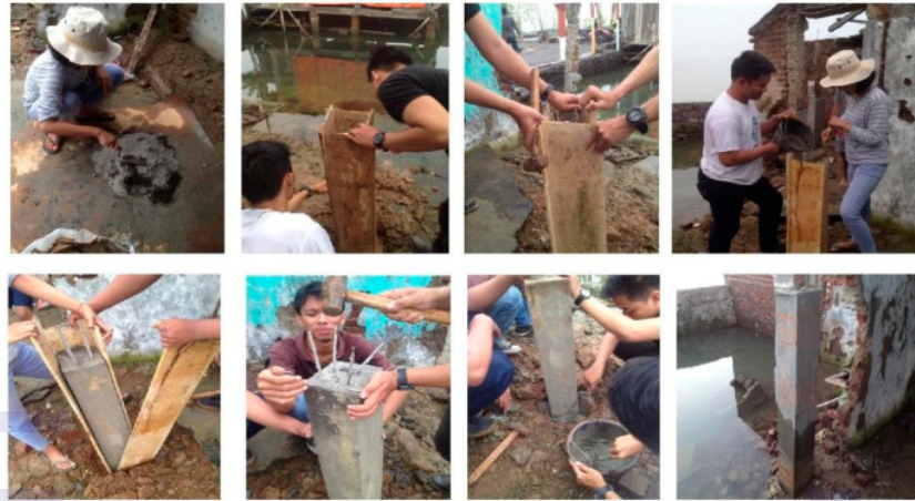
Figure 8. Construction of control column.
