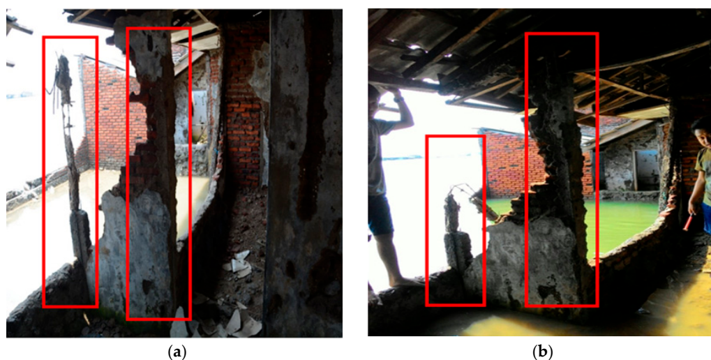
Figure 6. The broken columns which were retrofitted by applying bio-polymer modified concrete, (a) Situation at the time the left column still existed, and (b) Situation in the next few months after the left column had almost collapsed.
