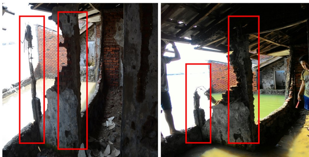
Figure 7: The broken columns which were retrofitted by applying bio-polymer modified concrete, (a) Situation at the time the left column still existed, and (b) Situation in the next few months after the left column had almost collapsed.
