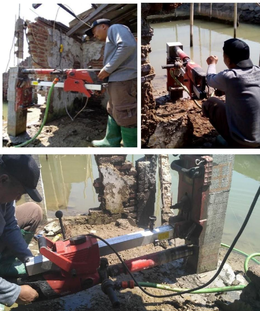
Figure 19. Core Drill method of retrofitted and control columns that was conducted to obtain samples which used for compressive strength test.
