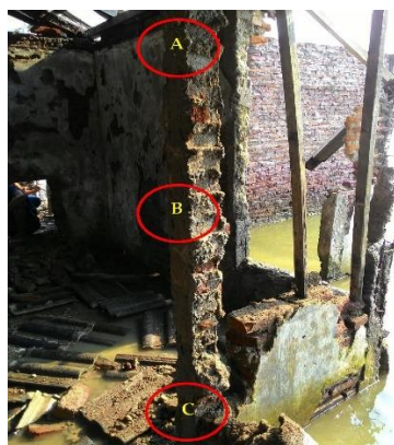
Figure 13. The Rebound Hammer Test was at conducted at the points that marked by red circles
