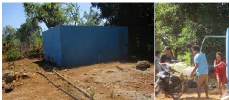
Figure 5. Public water reservoir of Government Project of PAMSIMAS [36]
