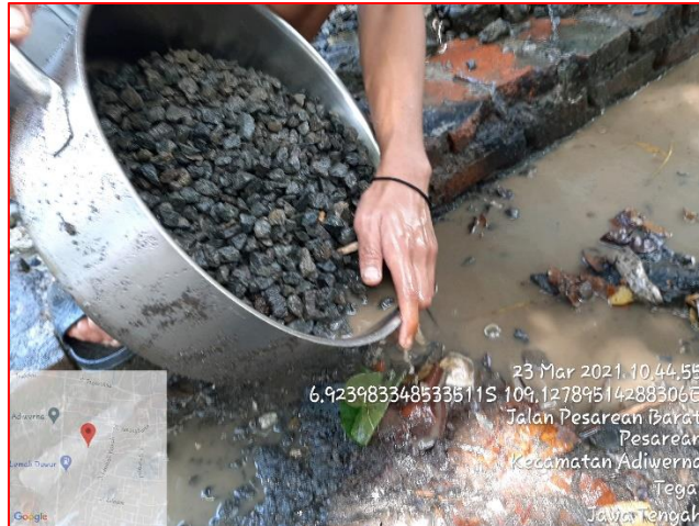
Agregat Kasar Splite
