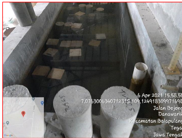
Proses Perendaman Beton
